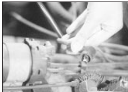
13.3 Inspect each HT lead end ferrule for corrosion
